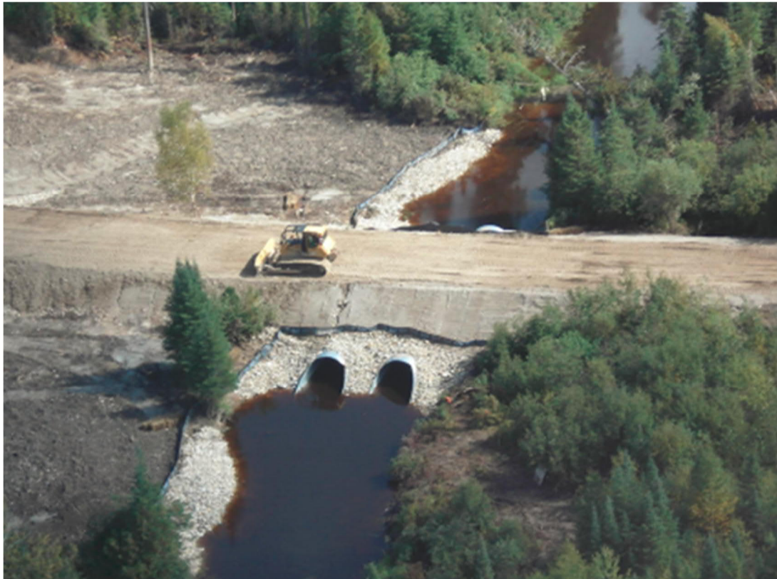
Figure 5-1: Fushimi Road – Fox River Culvert Construction
