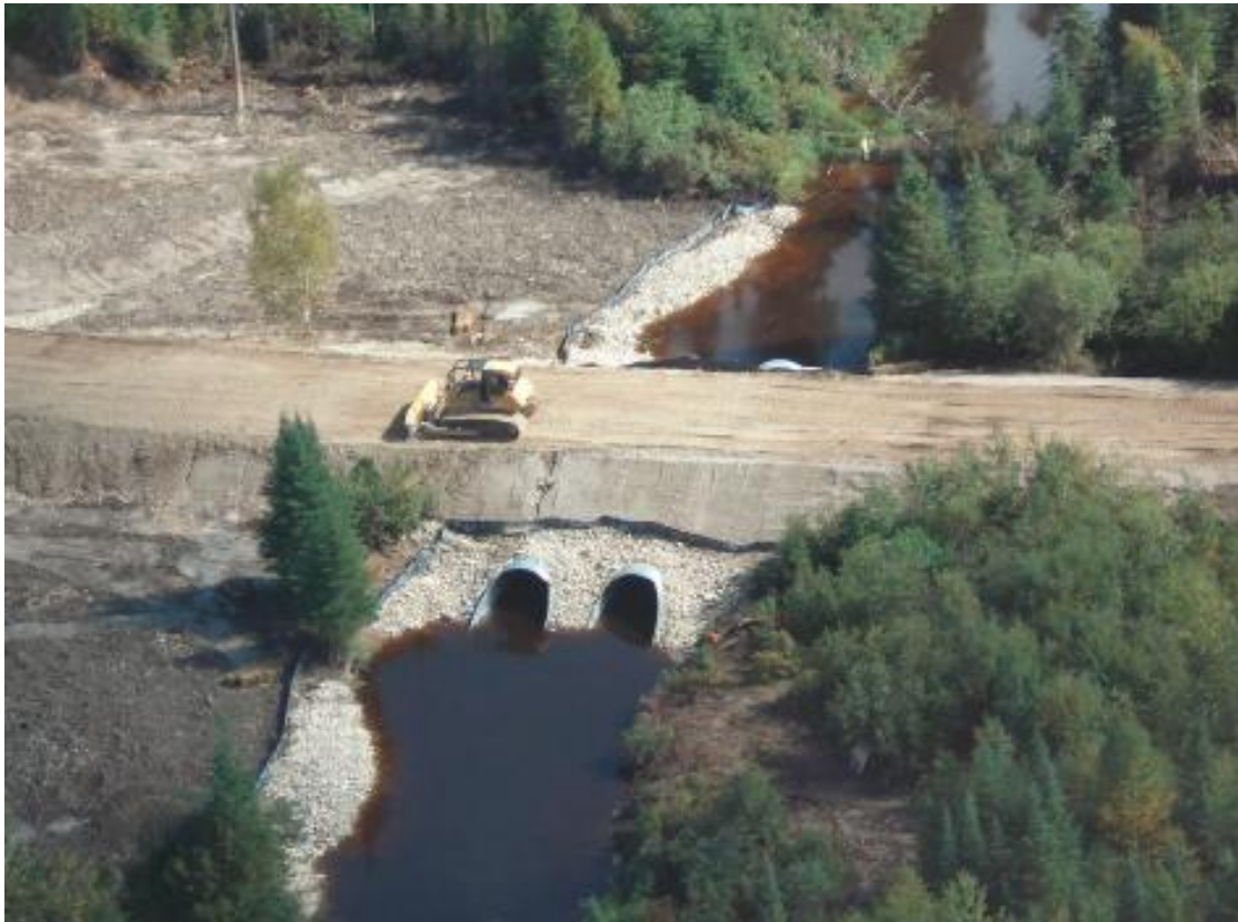
Figure 5-1 Fushimi Road - Fox River culvert construction
